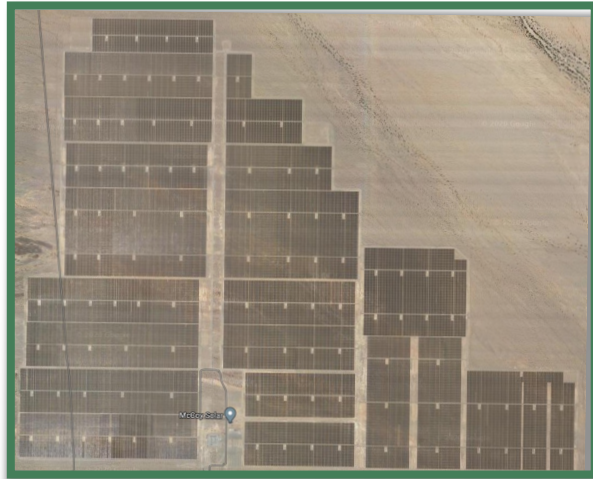
PV Power Plant (100s of inverters, 10s – 1,000 MW)
