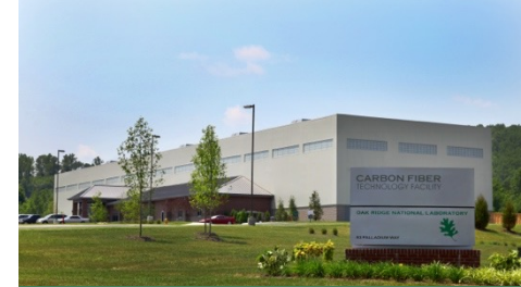
Carbon Fiber Technology Facility
